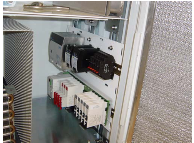
Opto 22's SNAP Ultimate I/O system installed in TrafficWerks ATPM.
