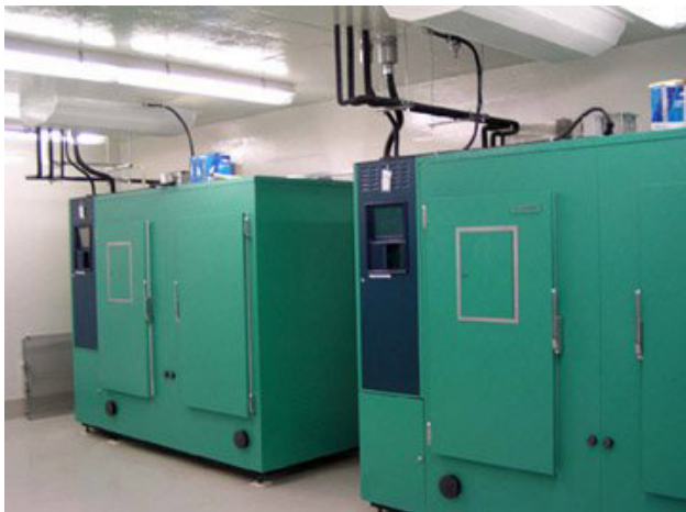
Energy consumption data from compressors and other equipment is acquired and sent to SQL databases.
