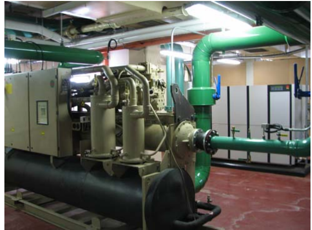
SNAP PAC controllers improve the overall performance of the heating, ventilation, and cooling system.
