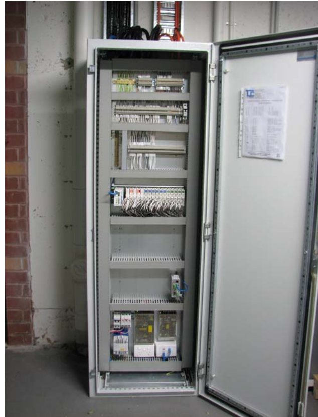
PID-maintained positive air pressure keeps airborne germs out of the operating room.
