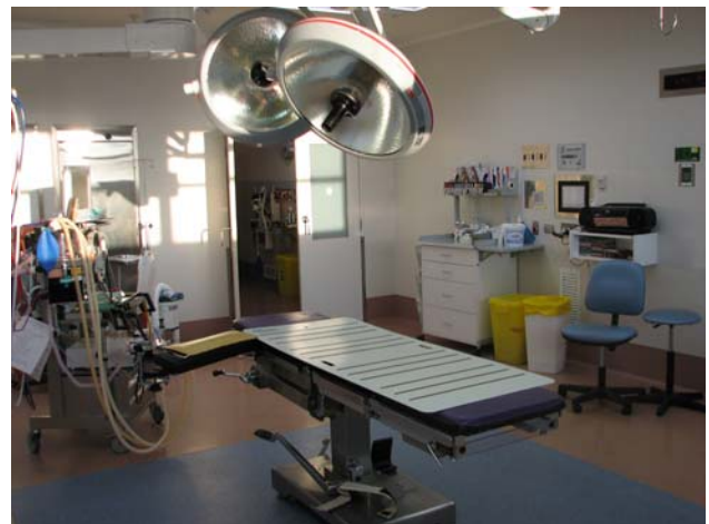
Wall-mounted OptoTerminal touchscreens allow doctors and nurses to adjust operating room temperature.
