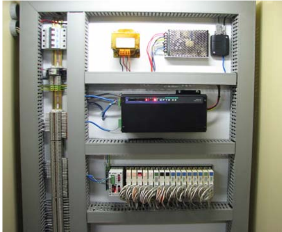
M4 controllers are replaced with SNAP PACs without having to touch any remote I/O or sensors.
