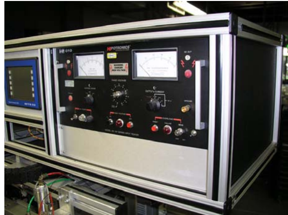
An embedded hi-pot machine applies voltage for many of the G4 modules' various tests
