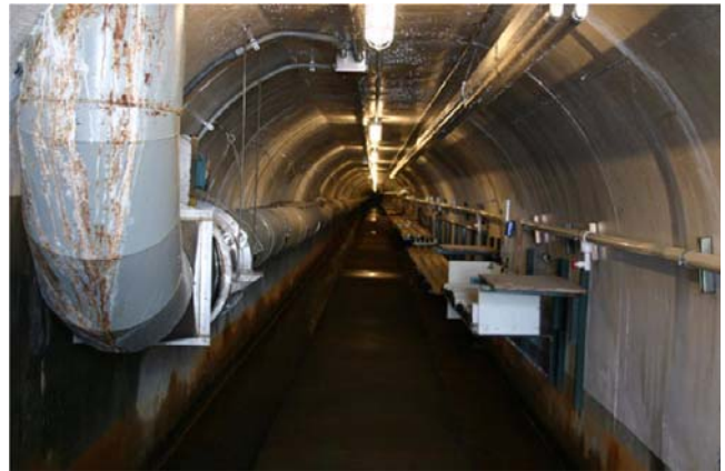
Interior of one section of the LMDT
