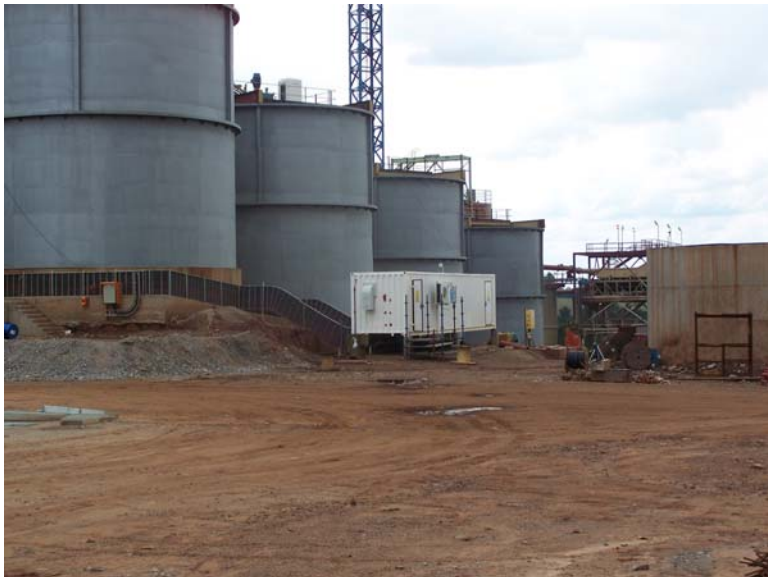
The Opto Controls control systems are located in large containers like this one in front of the large storage tanks.
