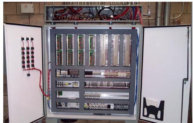
***The OptoEMU Sensor and other SNAP PAC System hardware is wired to SUPERVALU’s refrigeration system components and gathers consumption data. This data is then made available to both the company and curtailment service provider Net Peak.***
