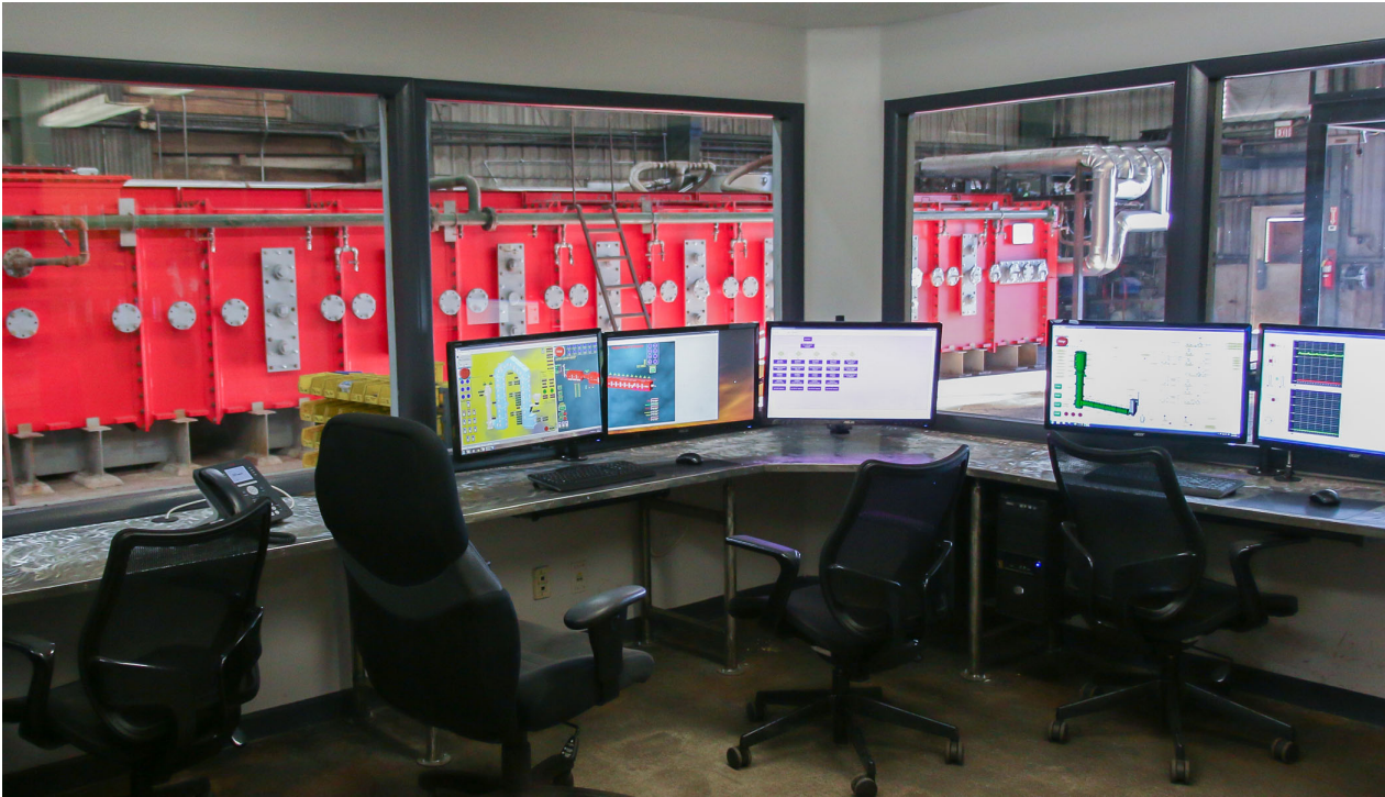
Figure 4: All operations of process equipment at IGRS can be monitored and controlled from this central control room.
