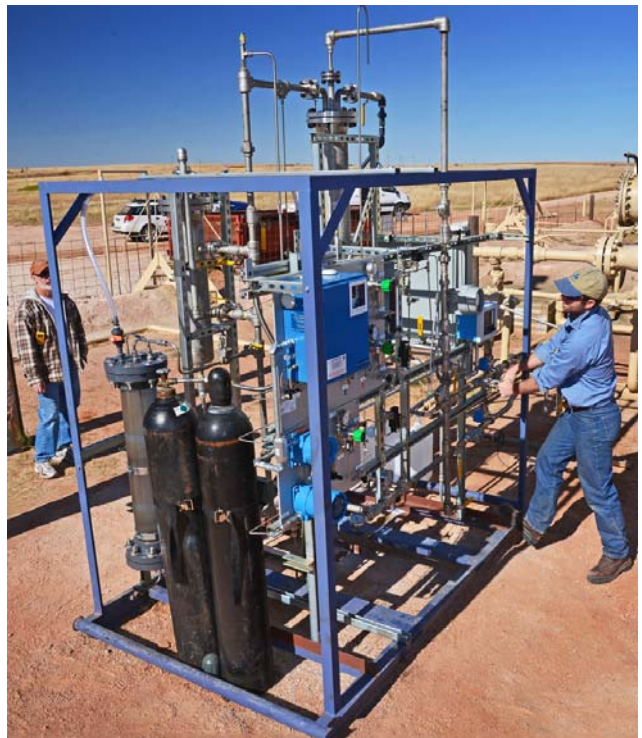
New Sky Energy's SulfurCycle natural gas scrubbing process is automated and monitored using Opto 22's SNAP PAC System control hardware and software.
