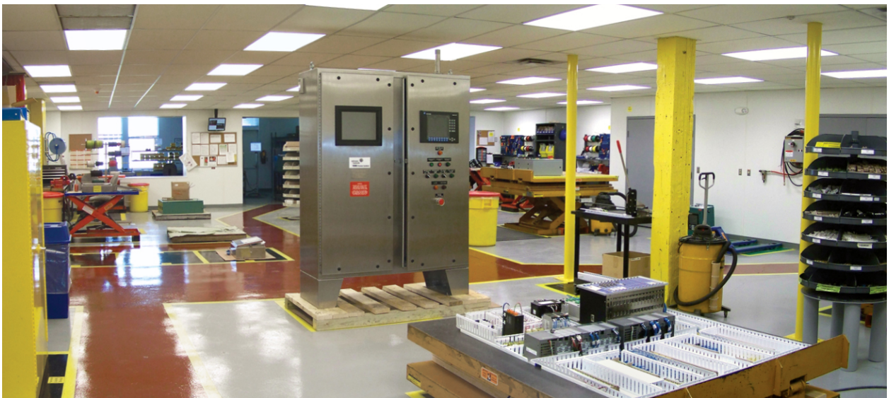
In this photo, Opto 22 control hardware is being added to a control panel. Frick Engineered Control Solutions builds on average 4000 panels per year.
