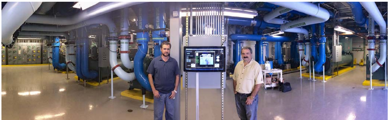
Carlos Terrazas (left) and Drazen Baricevic (right) with Arizona Facility Services (AFS) in the chiller plant of a retrofitted data center.
