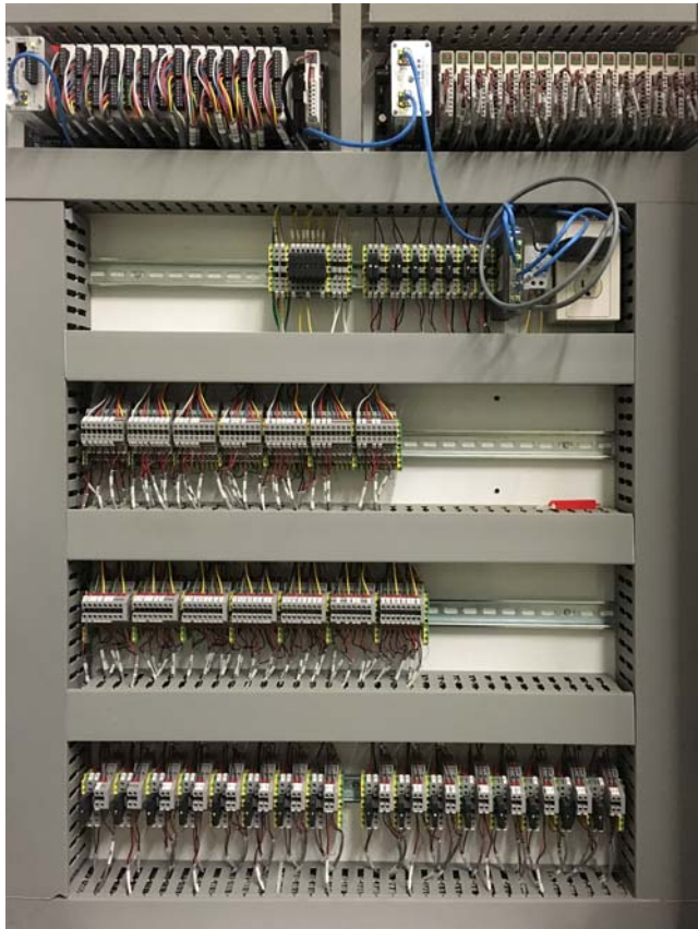
CalCA incorporates Ethernet-based Opto 22 control systems, shown here at the top of equipment deployed at a customer's location.
