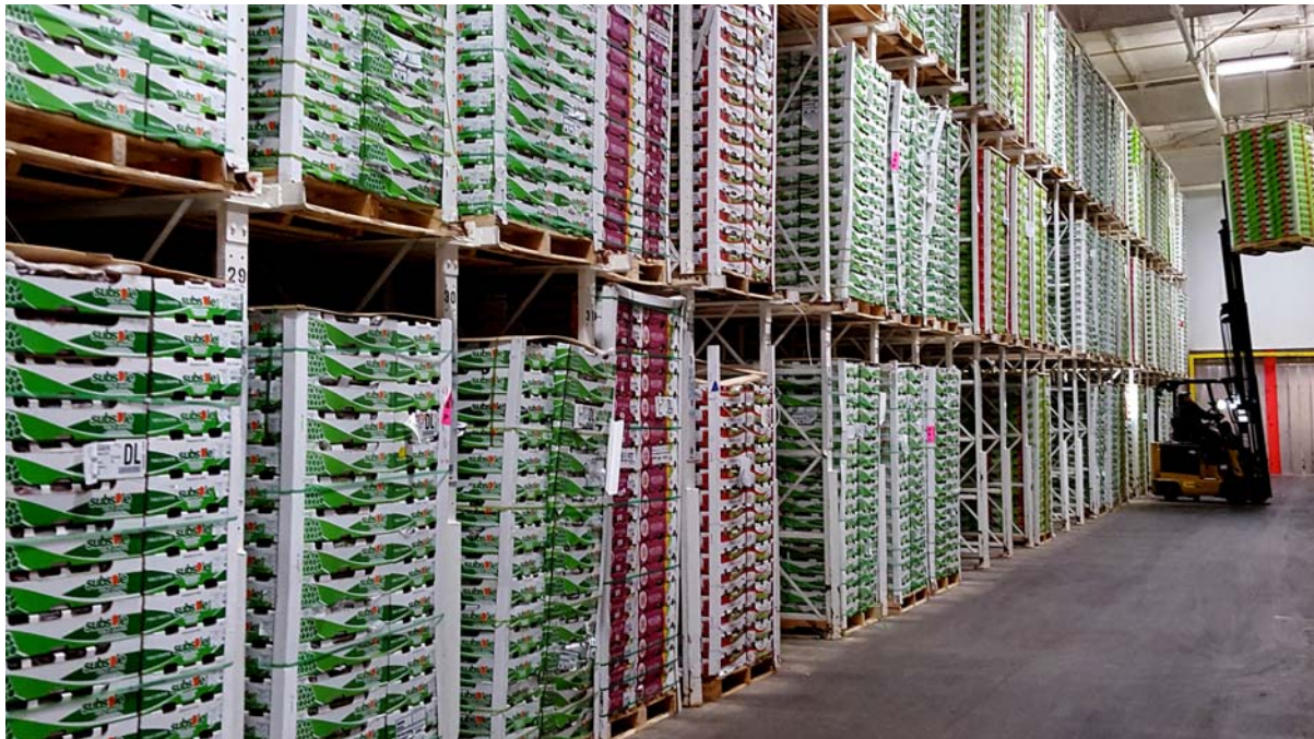
Controlled atmosphere storage rooms can store produce for months at low temperatures and oxygen levels.
