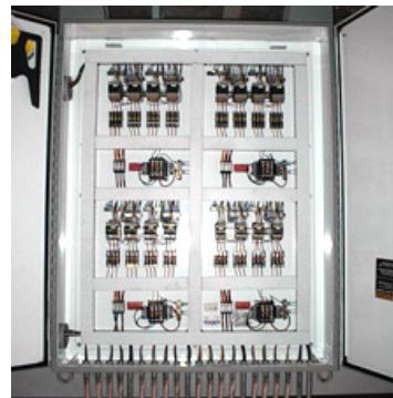
For energy efficiency, each of the five compressors has three stages of loading, providing exactly the amount of cooling required by the system. The control system also balances the run time of the various compressors by alternating the lead/lag relationships of each controller to ensure equal run time for all the units.
