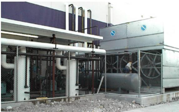
For efficiency, the same 170° Fahrenheit high-pressure refrigerant that cools the evaporators is also used in the defrost cycle for the evaporators.
