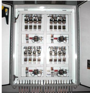
For energy efficiency, each of the five compressors has three stages of loading, providing exactly the amount of cooling required by the system. The control system also balances the run time of the various compressors by alternating the lead/lag relationships of each controller to ensure equal run time for all the units.
