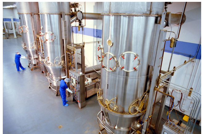
Storage Tanks (Outstations)
