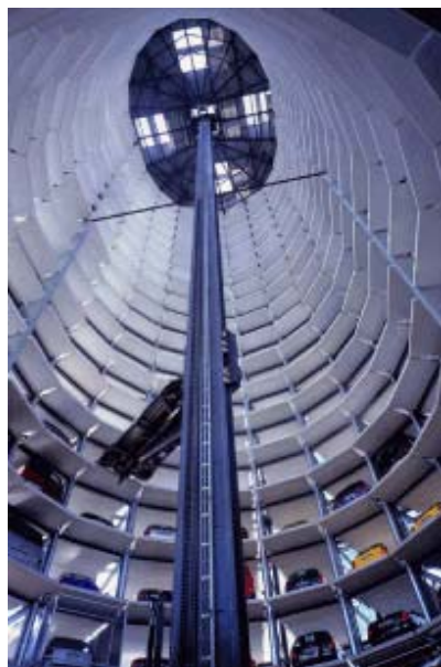
Figure 3: At Autostadt, taking ownership of your new car is an event in itself. In a fully automated procedure, your car is brought down to you from a 20-story car tower.
