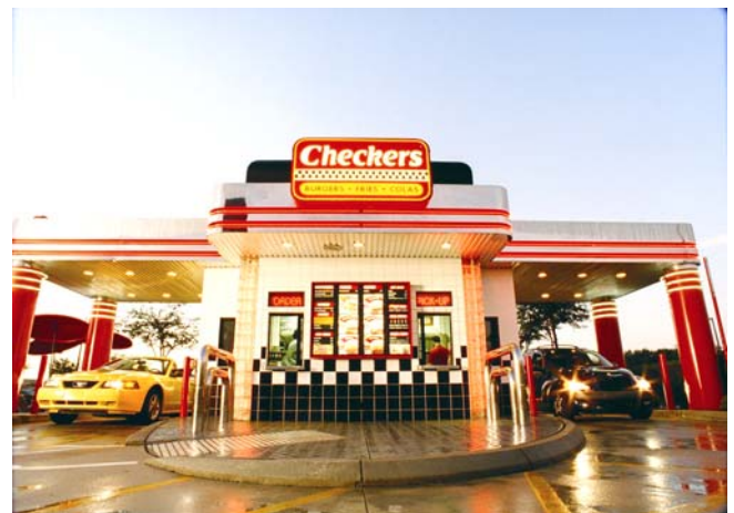
Checkers Two-Lane Drive-Thru
