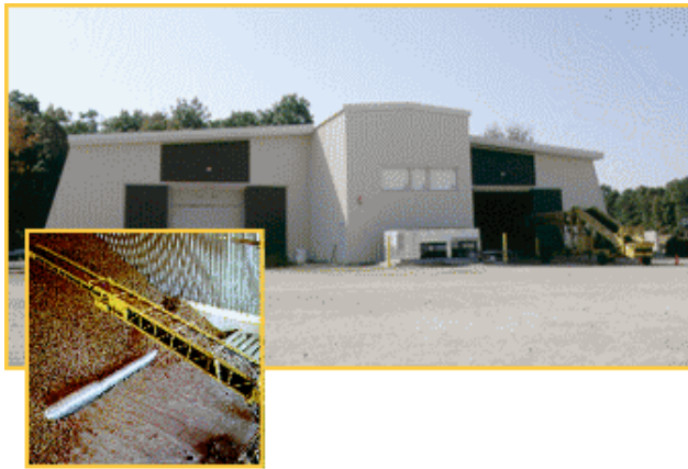
Rubber-belted conveyors move potatoes into Alsum's storage facilities which are environmentally monitored and controlled by the SNAP Ultimate I/O system.
