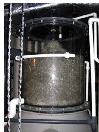
Dissolved organic compounds are collected at the tip of the protein skimmers and disposed of.
