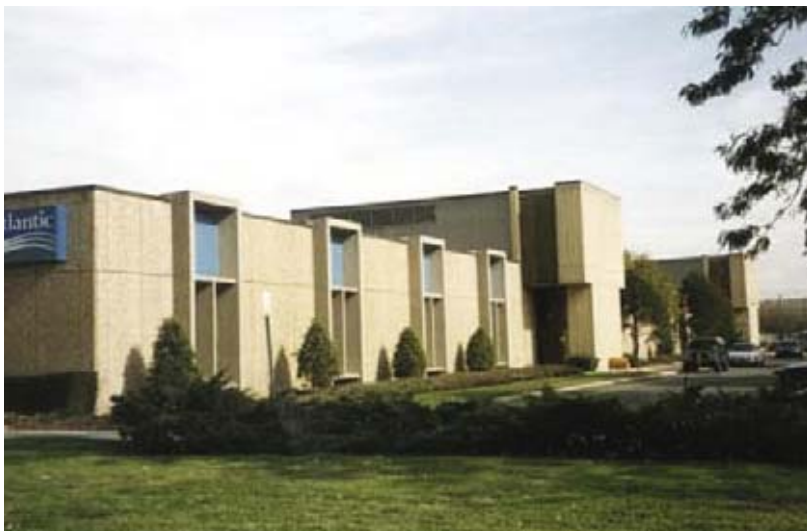
Verizon's "Central Office of the Future" in Garden City, Long Island
