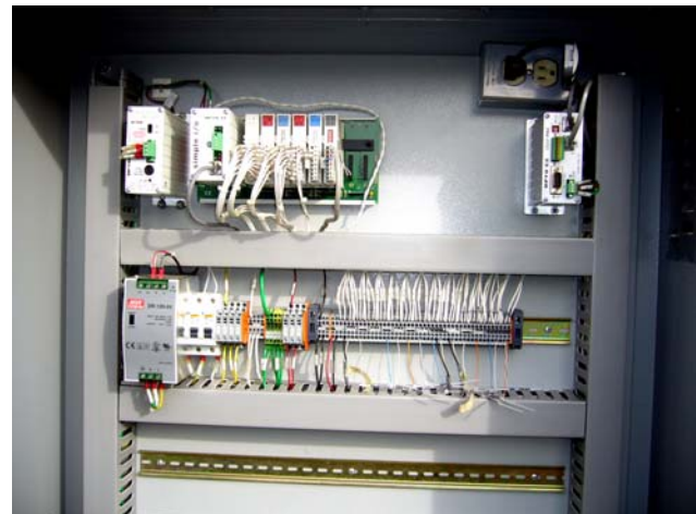
Opto 22’s SNAP Simple I/O System connects to Ecopetrol’s oil pumping equipment. The SNAP PAC (top right) controls the system.
