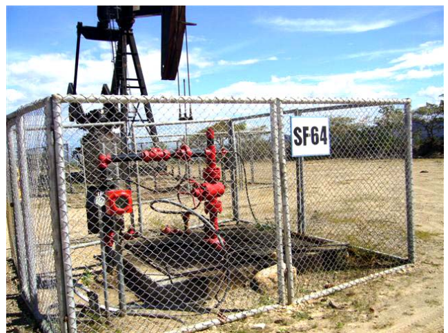
An Ecopetrol pumpjack
