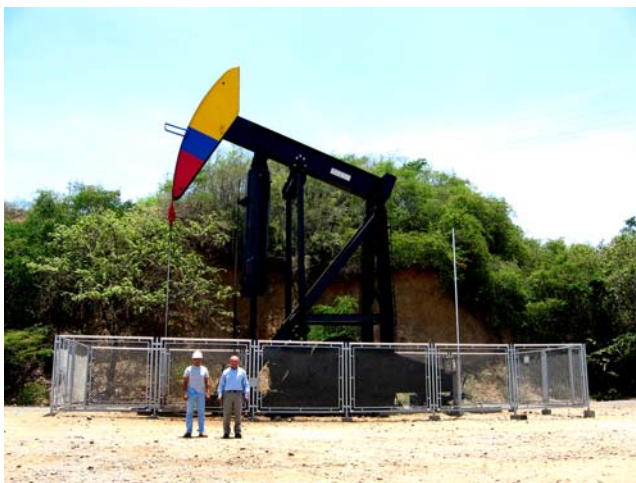
Ecopetrol pumping site
