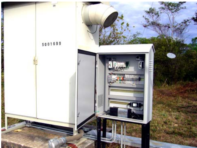
Opto 22’s SNAP Simple I/O System connects to Ecopetrol’s oil pumping equipment. The SNAP PAC (top right) controls the system.
