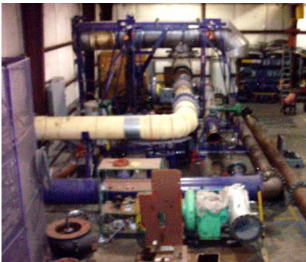
The NGML uses a unique closed-loop design, allowing for complete testing of the turbocharger compressor and turbine over the entire operating range.
