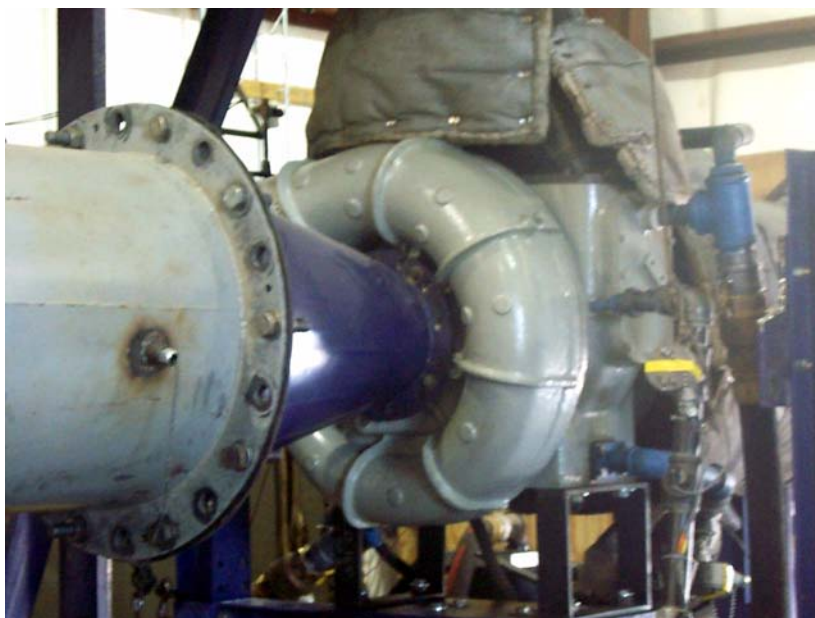
The NGML contains a large assortment of resources to conduct a full battery of mechanical, performance, and load line tests.
