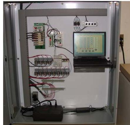
*Opto systems manage tank water temperatures, water flow and oxygenation, and equipment status*
