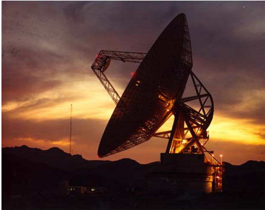
In Madrid, an antenna similar to this one will be equipped with load cell transducers and the SNAP PAC System to discover why cracks have developed in the large elevation bearing system.
