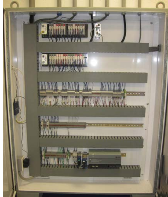
Before and after: The photo above shows the original plant wiring. At right, the ISI-built control cabinet with Opto 22 SNAP PAC hardware.
