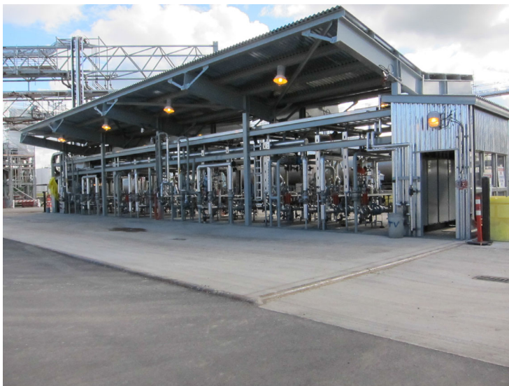
A loading rack for tanker truck transfers
