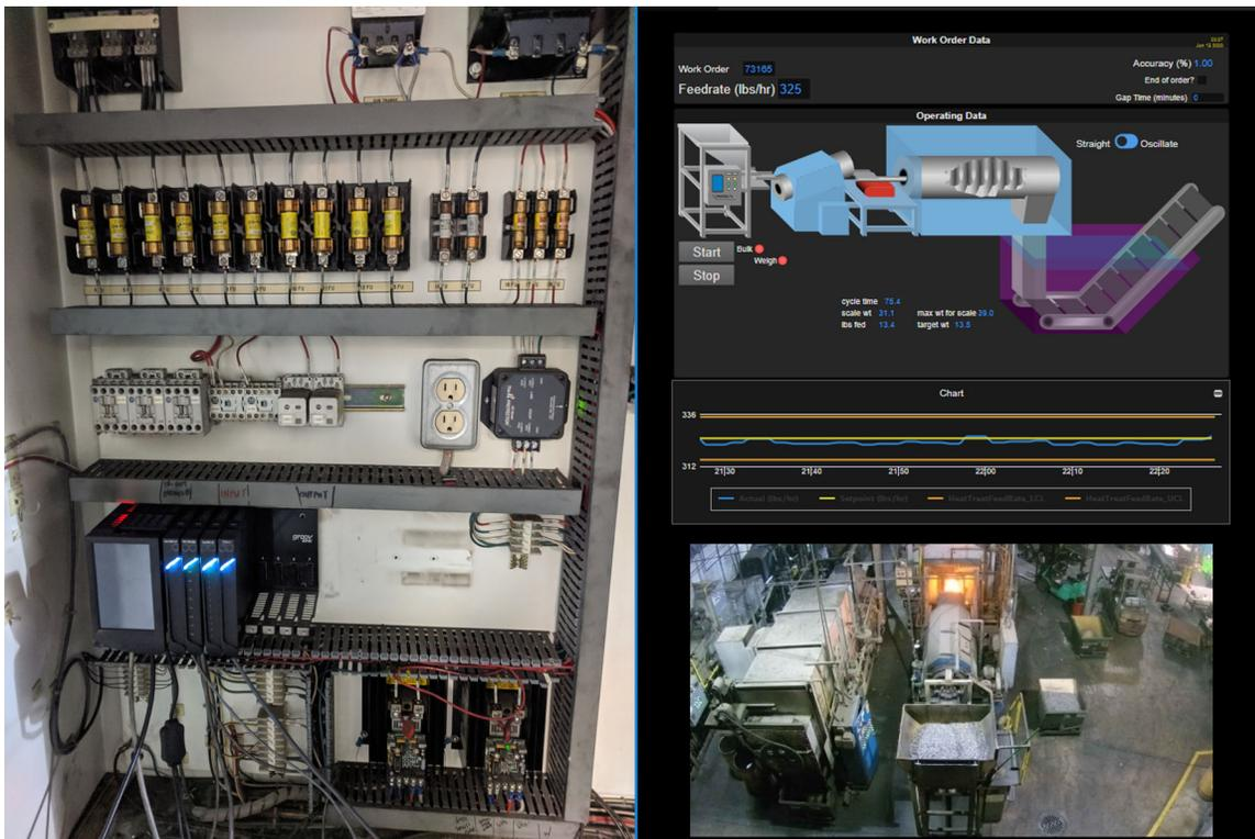
New electrical panel layout with *groov EPIC* and accompanying *groov View* HMI
