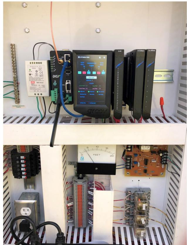
A comparison of one of Waterford DPW’s lift station control panels showing the old RTU layout and the new layout with the *groov* EPIC controller and DIGI modem.
