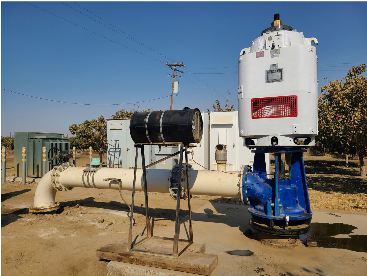
Azcal well pumps all feed the same mainline pipe, leading to complex pressure management requirements.
