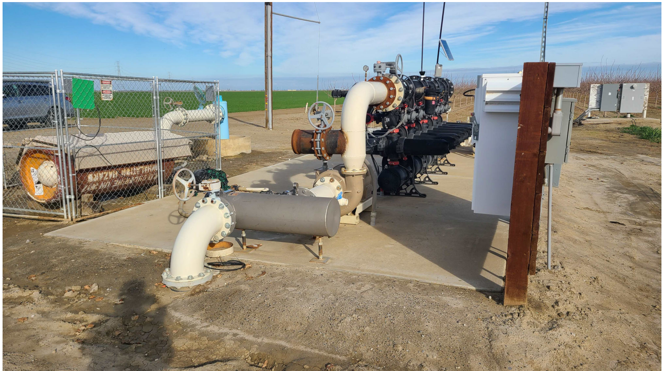
All Azcal wells and irrigation filter stations are equipped with VFDs and flow meters.
