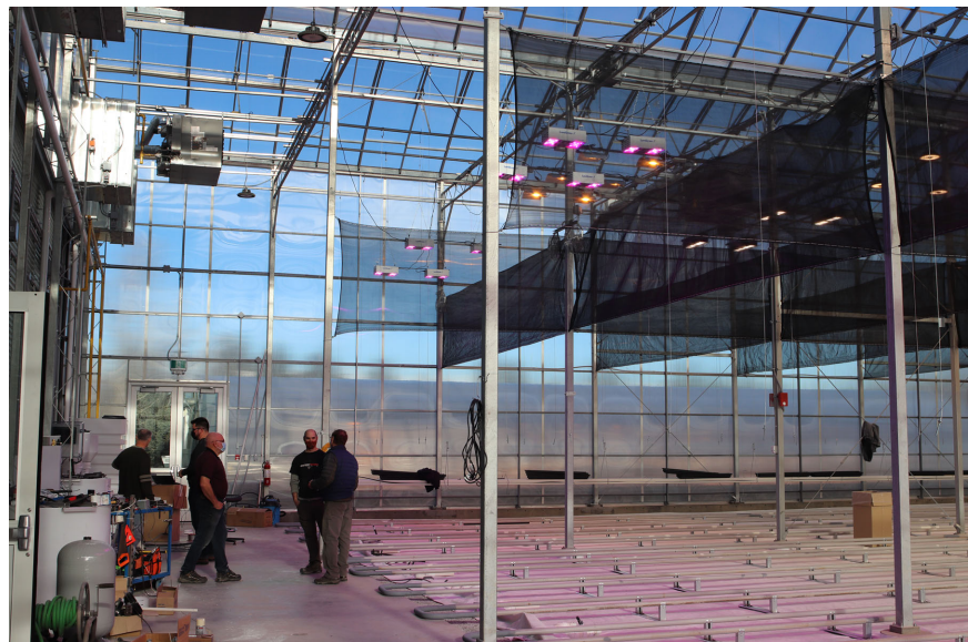
The Aquaculture Centre of Excellence greenhouse under construction
