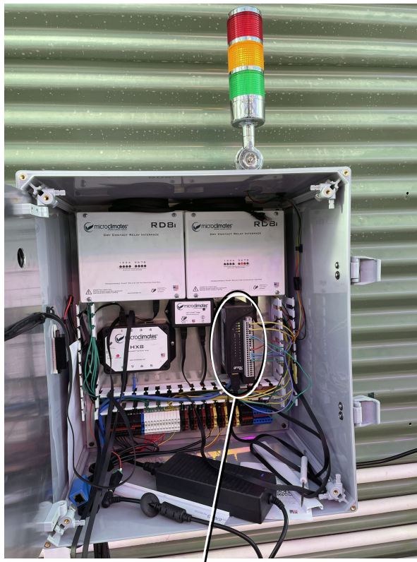
The groov RIO (circled) connects to sensors, provides cybersecurity features, and runs the Microclimates software.
