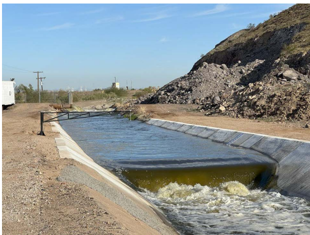
Gila Bend main canal at Gillespie Dam
