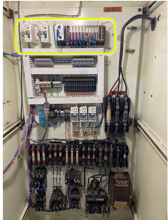
Mercer's older systems, still running reliably, use an Opto 22 SNAP PAC System.
