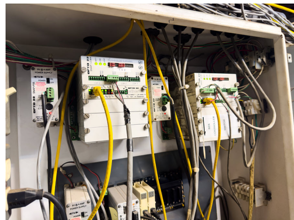
Varland Plating's legacy Opto 22 SNAP-LCM4 controllers
