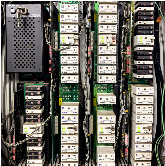
Varland Plating's legacy Opto 22 mistic analog racks
