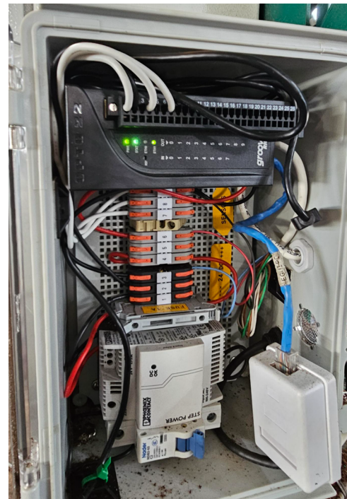
A counter system using the groov RIO
