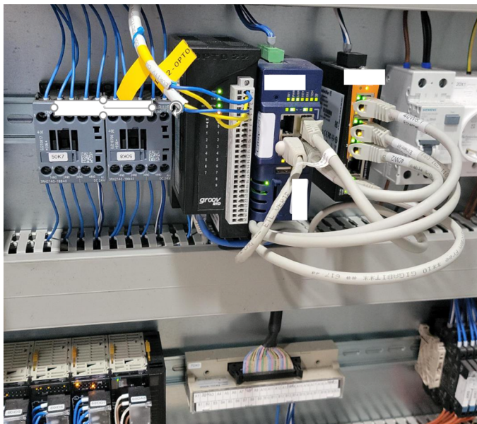
Using groov RIO to bridge the communication gap
