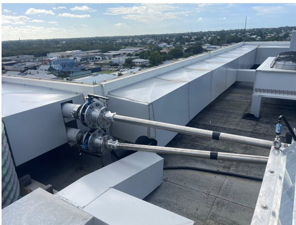
Rooftop views: new radiator pipes connected to existing copper pipes
