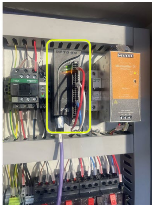
groov RIO EMU tracks power conditions to ensure stable generator operation.
