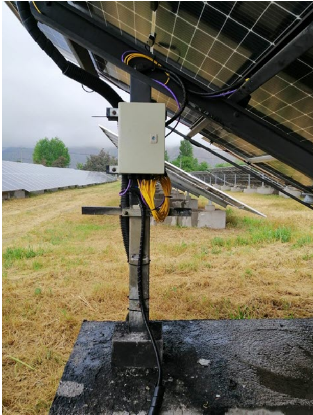
Field-mounted junction box on a solar panel in the photovoltaic array
