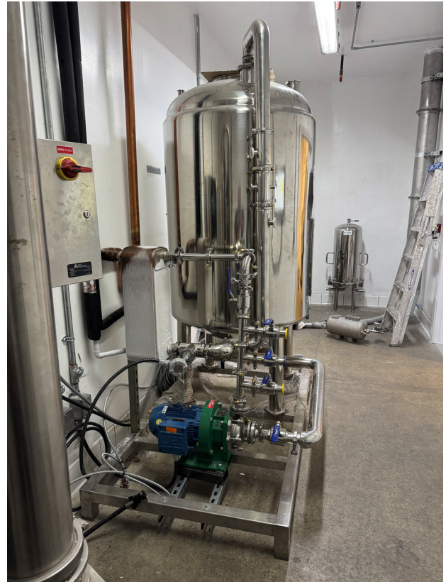
PermaCool's stainless steel chiller assembly integrates precision pumps, valves, and heat exchangers to maintain consistent process temperatures.
