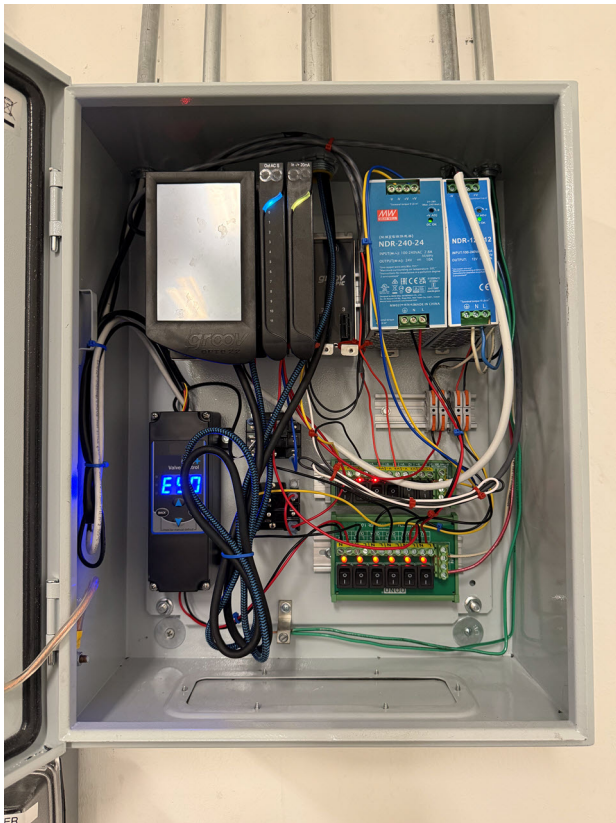
In-house control panels with the groov EPIC system combine processing, networking, and I/O in a single compact enclosure
