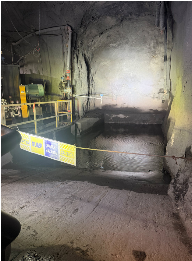
An underground sump pump station containing a motor, discharge piping, and staging platform with a water hazards barrier
