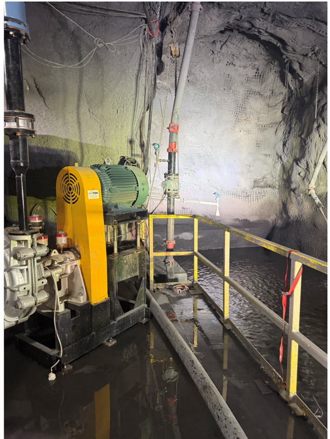
An underground sump pump station containing a motor, discharge piping, and staging platform with a water hazards barrier
