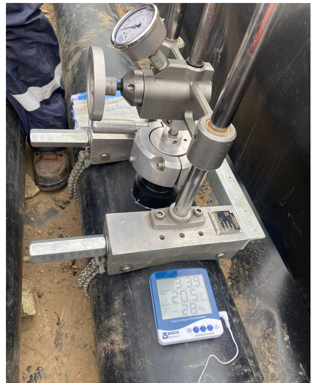
Validating pipeline measurements
