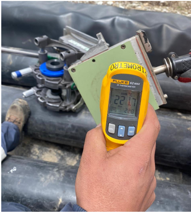
Taking pipeline measurements
