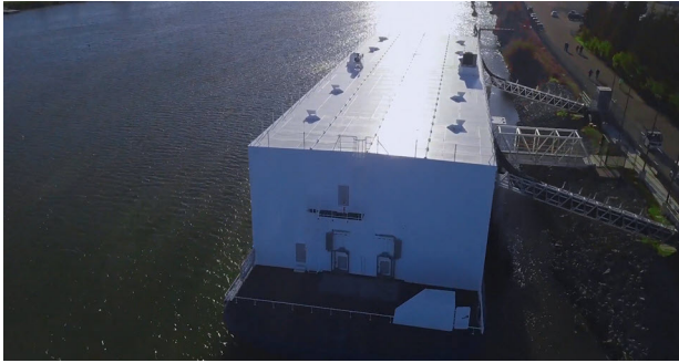
River water cools the Nautilus floating data center.
