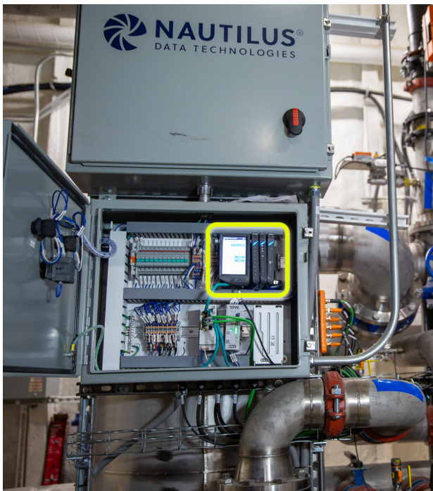
Opto 22's groov EPIC provides the control solution needed in the EcoCore FCD.
