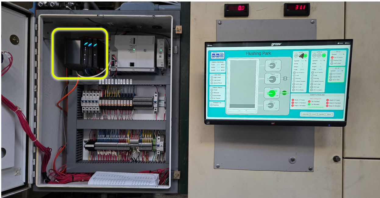
groov EPIC running local control and I/O, with groov View providing a live operator interface while data is shared via Sparkplug B MQTT.
